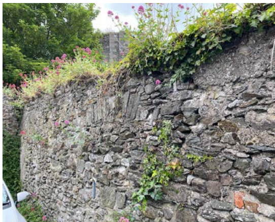
31. Detail of infilled door head in wall along lane.
