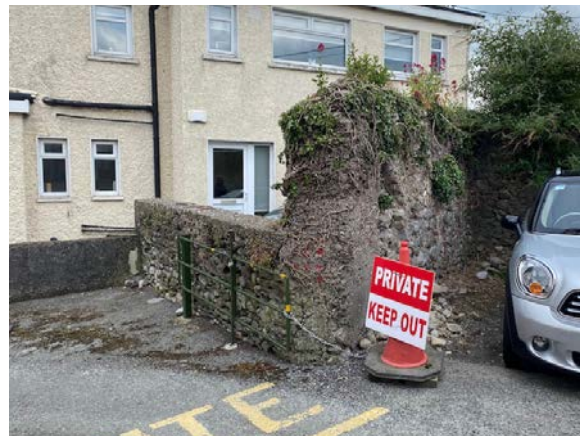
49-51. Views of wall fragments to rear of Abbey Road.
