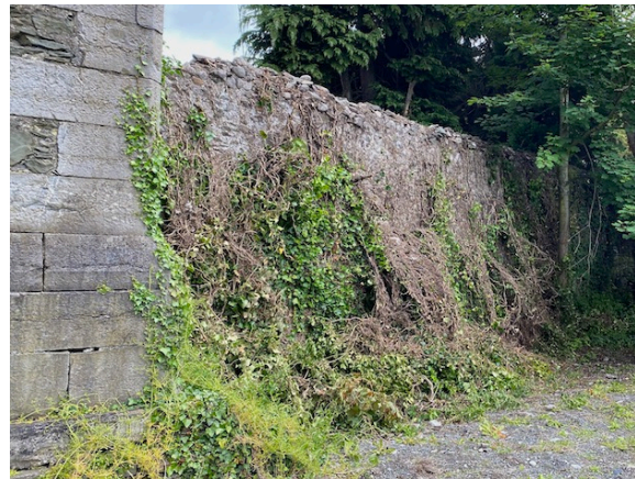
29. View of boundary wall to church and base of tower.
