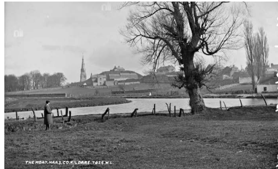
6. Photograph over canal towards North Moat ca.1900 (NLI).
