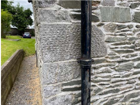
42. Detail of medieval punched stonework to church.
