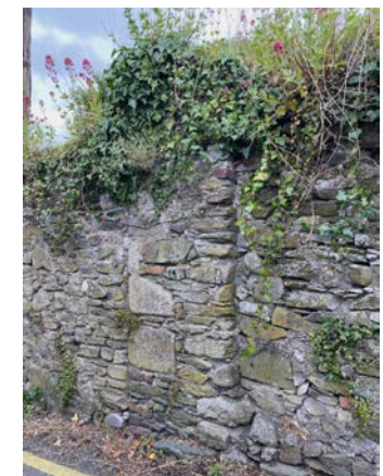
34. View of pier of former structure along lane.
