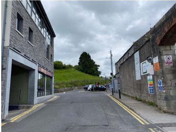
21. View along Abbey Street towards the North Moat.
